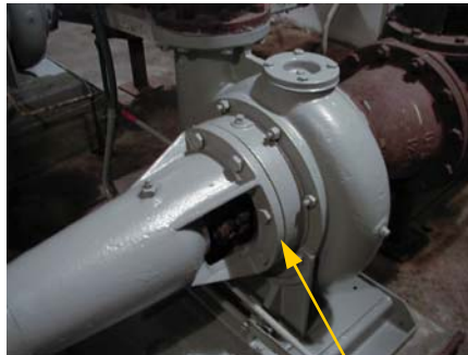
FIGURE 1: PUMP SLEEVE AS SHOWN IN SERVICE
